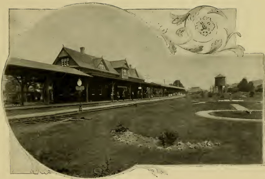
DELAWARE, LACKAWANNA & WESTERN STATION, STROUDSBURG, PA.
